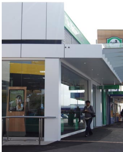
National Bank Blockhouse Bay.
