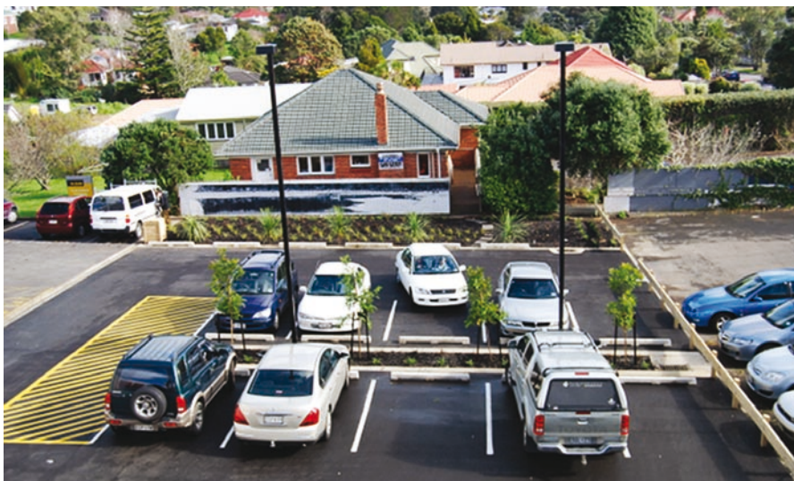
Features outside the building include the planting to shade vehicles and the rain garden at back of car park with compost bin.
